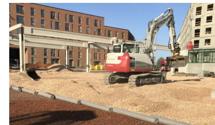
The system build-up is designed for high loads and can be driven over by excavators.
